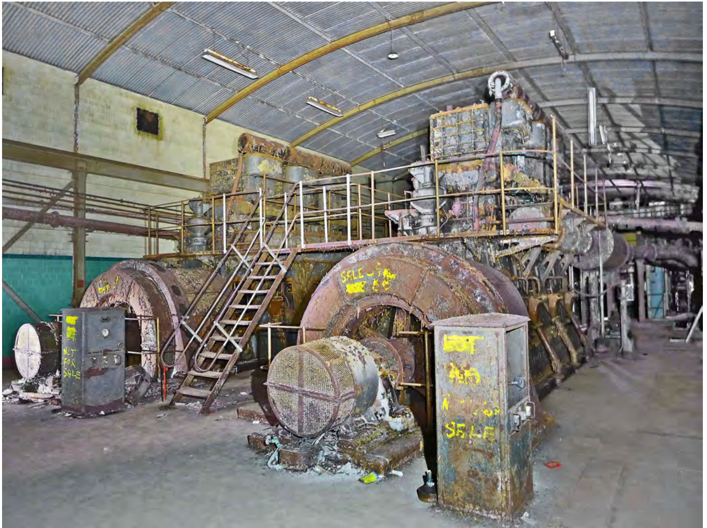
Calpe Hole generating station: two of the English Electric Fullagar diesel engines and generator sets
